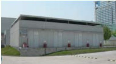
Hazardous material warehouse with double roofing
