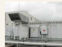
Fujinomiya factory: Catalytic oxidator
