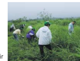
Progress of undergrowth cutting
