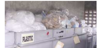
Storage space for plastic waste to be recycled
