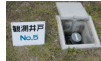
Observation well (Kofu Factory)
