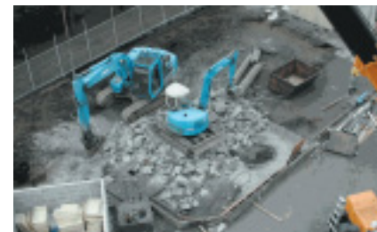
Incinerator being removed (removal of base)
