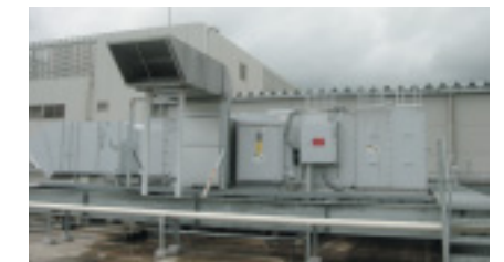
Catalytic filter-type waste gas treatment facility (Fujinomiya Factory)
