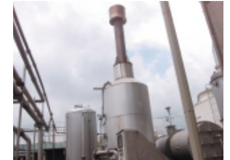
Incineration-type waste gas treatment facility (Ashitaka Factory)
