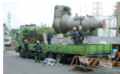
Incinerator being removed (transporting waste gas treatment facility)
